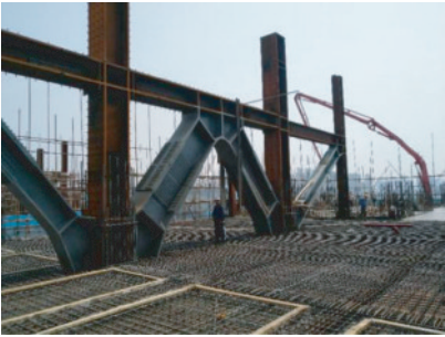
图2 转换层桁架施工现场照片 Fig.2 Photo of construction site of conversion floor truss
